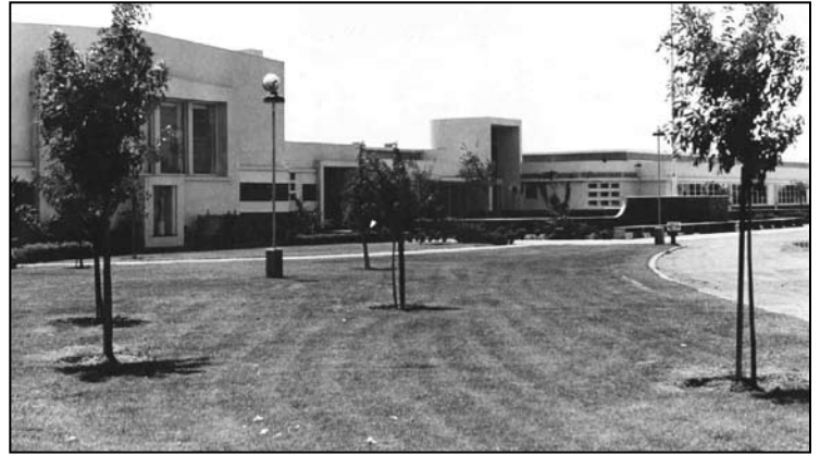
LAKESIDE ELEMENTARY SCHOOL
