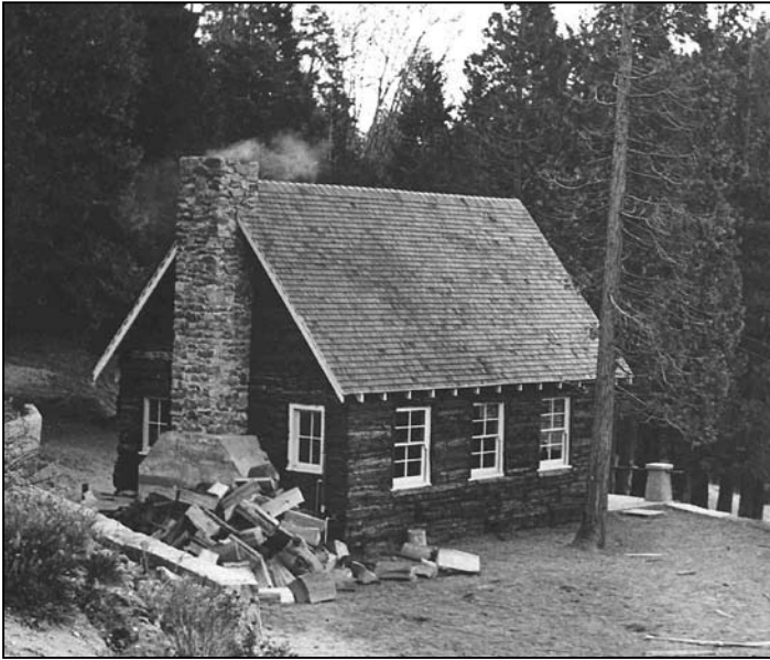
GREENHORN EMERGENCY SCHOOL
